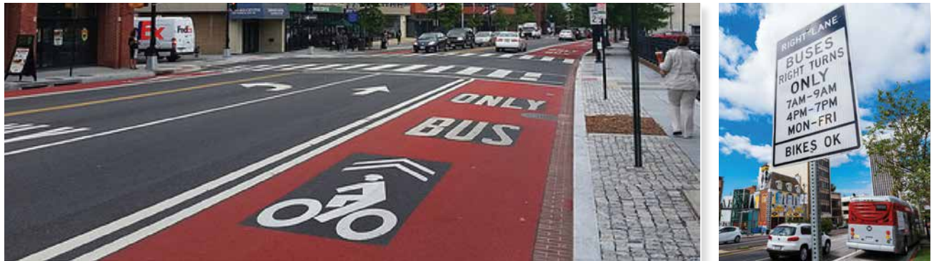
Figure C6.1: WMATA Peak-Hour Bus Lane on Georgia Avenue (shared with bicycle, left) & LA Metro Peak-Hour Bus Lane on Wilshire Boulevard (right)
