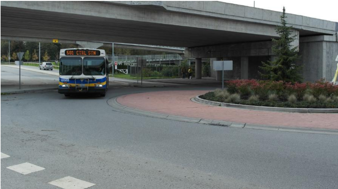
Figure 2.8.1 Example of roundabout
