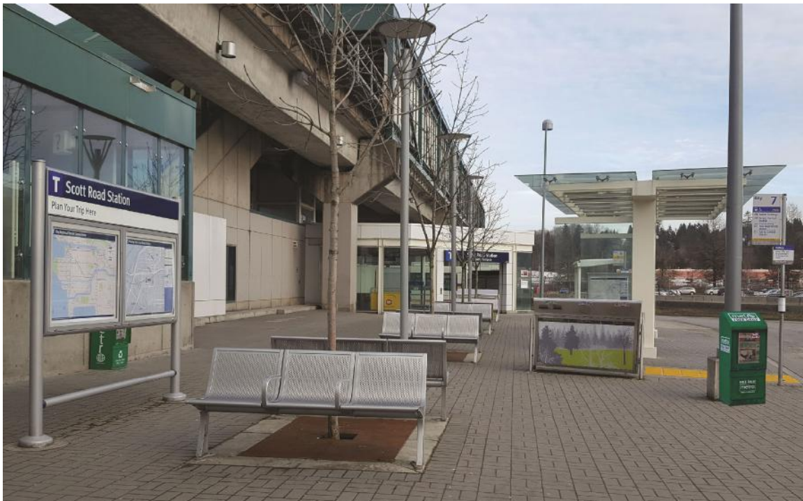
Figure 4.2.23 Scott Road Station Transit Exchange amenities
