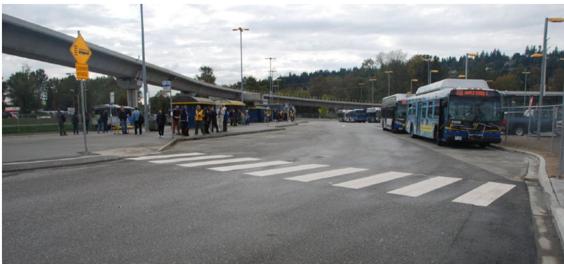
Figure 4.2.14 Example of pedestrian crossing within a transit exchange at Coquitlam Central Station
