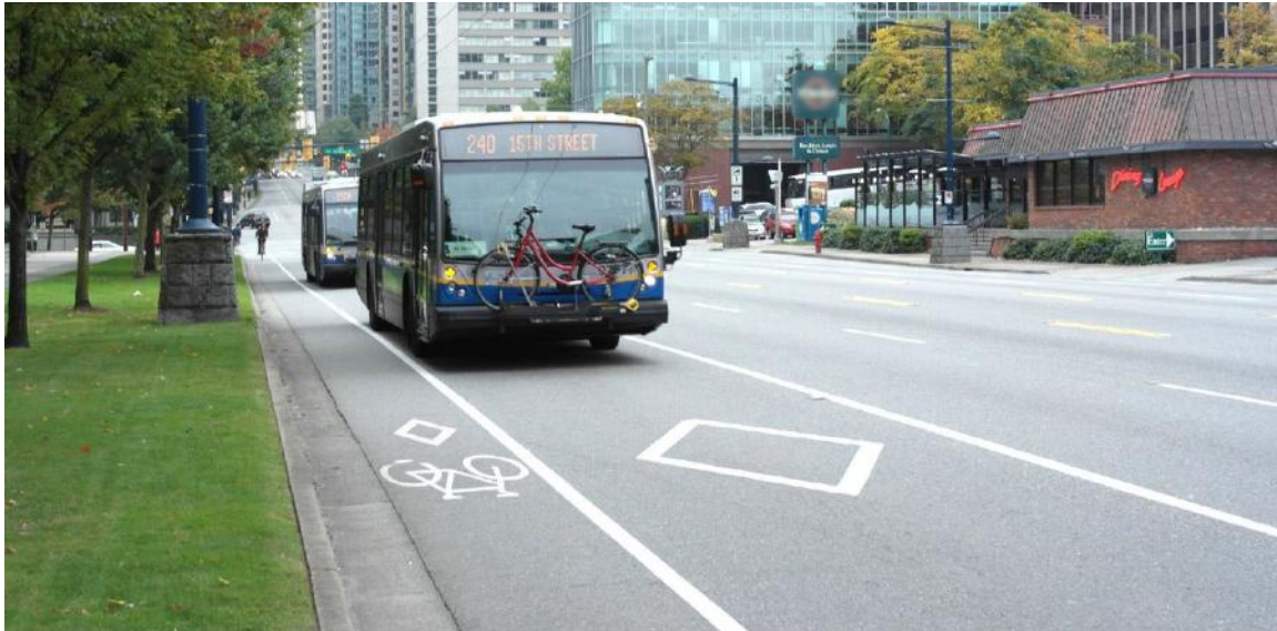
Figure 5.2.2 Example of bus-only lane (West Georgia Street)
