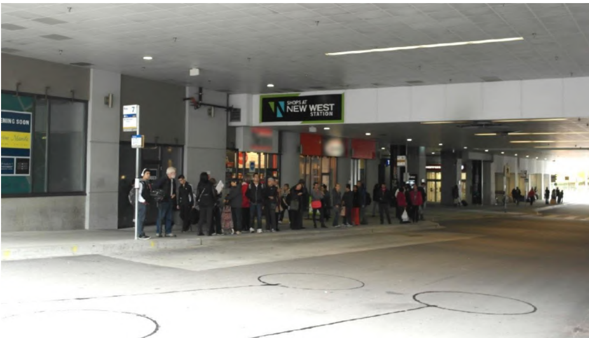
Figure 4.2.19 New Westminster Transit Exchange covered facility
