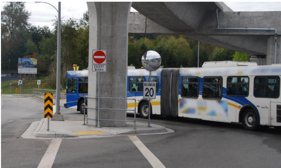
Figure 6.2.2 Entry prohibited sign
