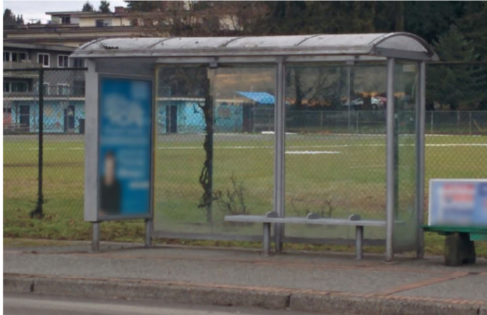
Figure 3.5.9 Example of a bus shelter
