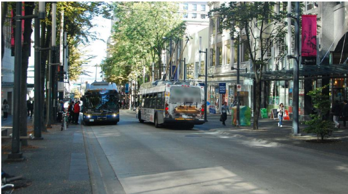
Figure 4.2.10 Granville Street (bus mall)
