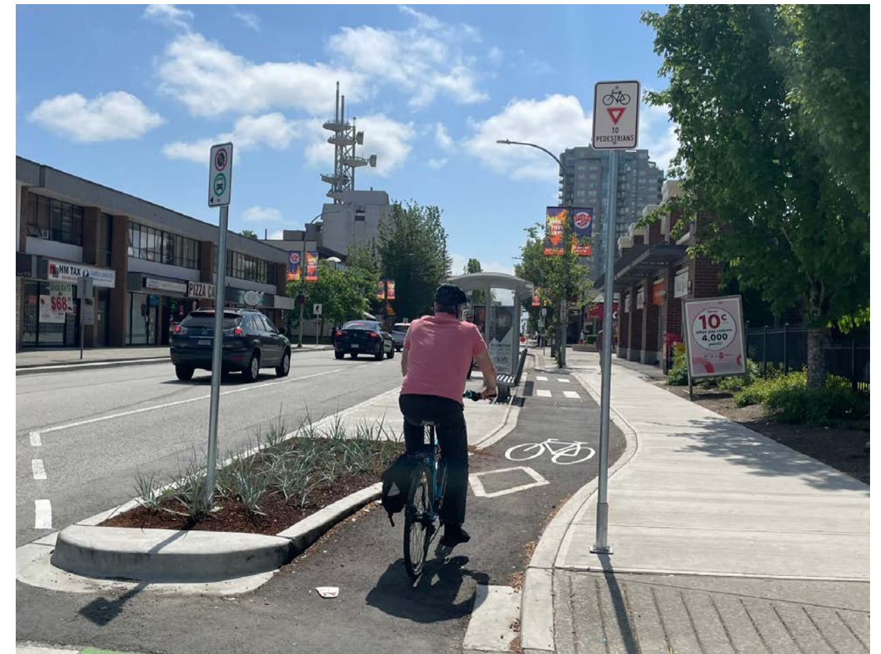
Figure 10: Colour Contrast Between Bikeway, Sidewalk, and Island Platform, New Westminster, British Columbia
