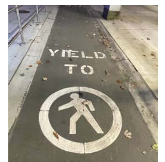
Figure 34: Example of Bicycles Yield to Pedestrians pavement markings, North Vancouver, British Columbia
