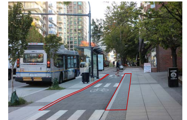
Figure 31: Examples of Edge Treatments that are Not Reliably Detectable, Burnaby, British Columbia (left) and Vancouver, British Columbia (right)
