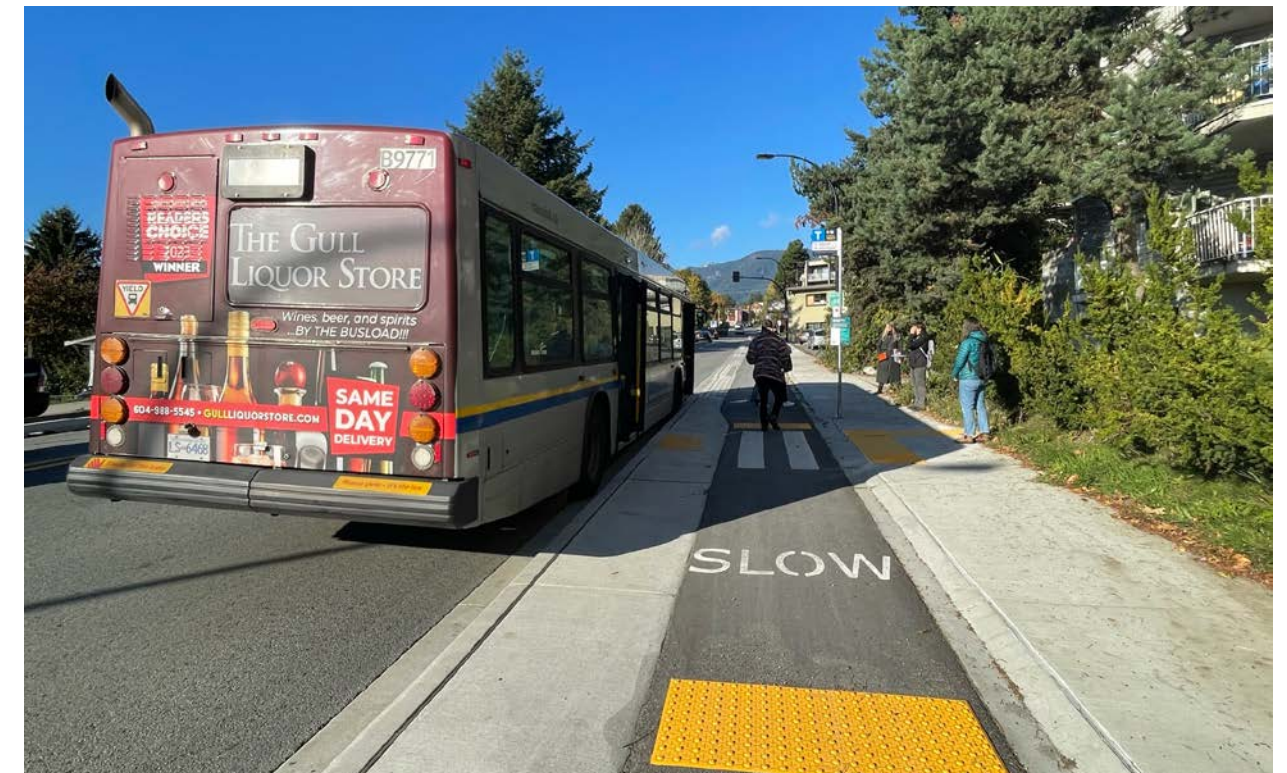
Figure 13: Detectable 'Bookend' in a Constrained Application Without an Island Platform Using Tactile Attention Indicators, North Vancouver, British Columbia
