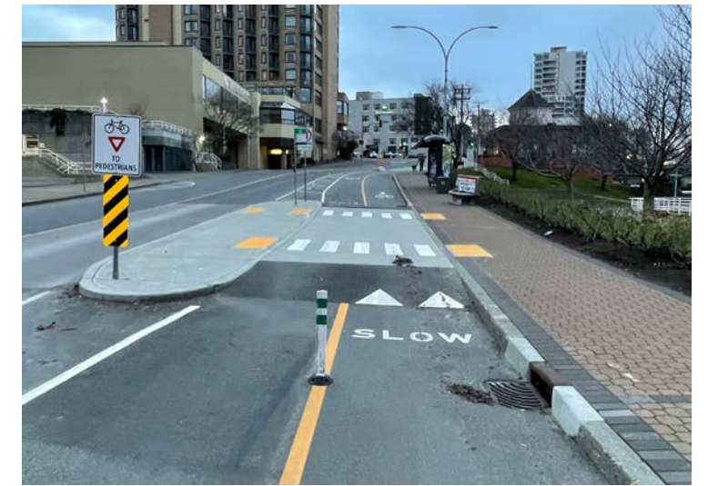
Figure 24: Bikeway Raised to Sidewalk Level Adjacent to Island Platform, Nanaimo, British Columbia
