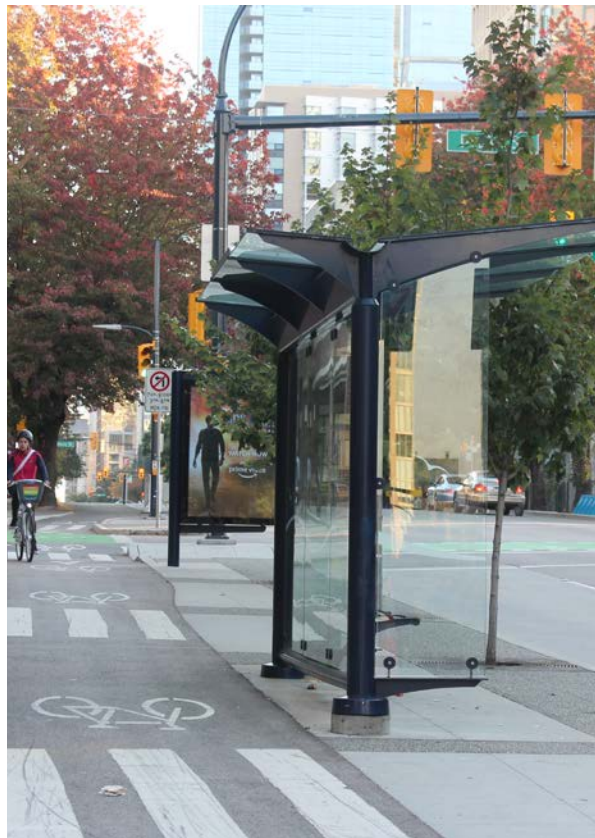
Figure 40: Example of a Bus Shelter with Clear Side and Back Panels, Vancouver, British Columbia
