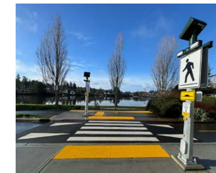
Figure 38: Actuated Flashing Beacon at Island Platform Crosswalk, Saanich, British Columbia
