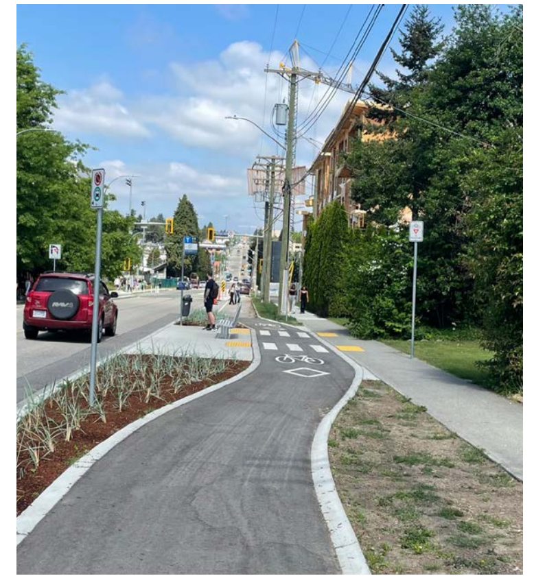
Figure 25: Horizontal Deflection of Bikeway Adjacent to Island Platform, New Westminster, British Columbia
